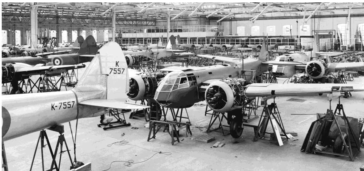
Above: Filton Blenheim Mk.1 production on 7 th June 1937; the prototype K-7557 with a slender rear fuselage can be seen in the left foreground, just behind is BL-104, the first aircraft for Finland which would wear a pale-blue swastika when in service. The rest of the RAF aircraft are first batch and have tail serials around K-7050; somewhere in the melee is also the first aircraft for Turkey.
